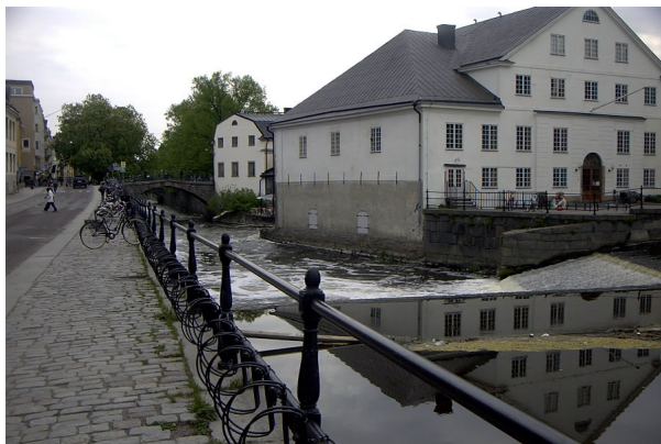
45. Uppland Museum is the white building in the foreground.
